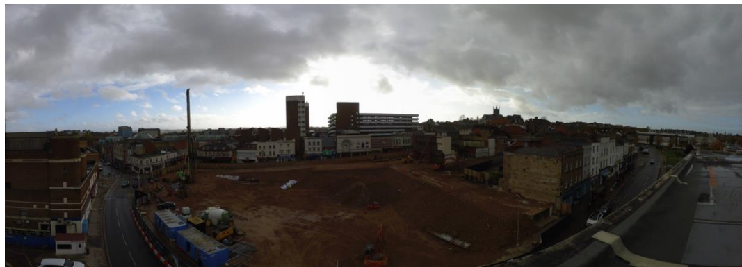
Figure 3 Time lapse image of Union Yard demolition works
